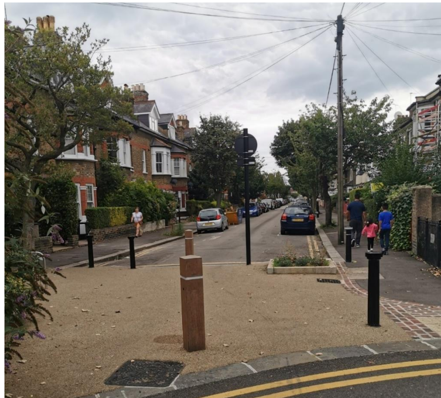
Figure 4-40: Modal filter removes through traffic, allowing walking and cycling and improving public real (Credit – Create Streets)
