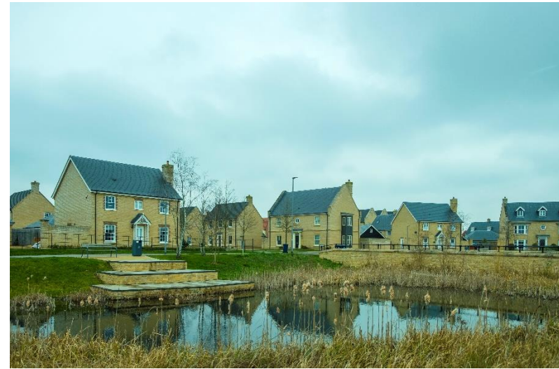
Figure 8-9: Attenuation pond acting as a focal point for adjacent homes, Alconbury Weald (Credit - Create Streets)
